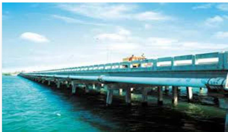
Slika 7. Boca Chica Bridge, FL.
